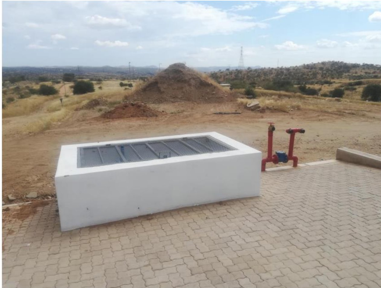
Fig 21: Showing a recently completed underground water storage tank and firefighting infrastructure
